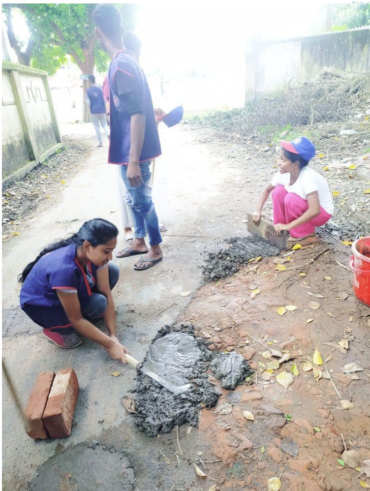
Repairing Road in front of the college
